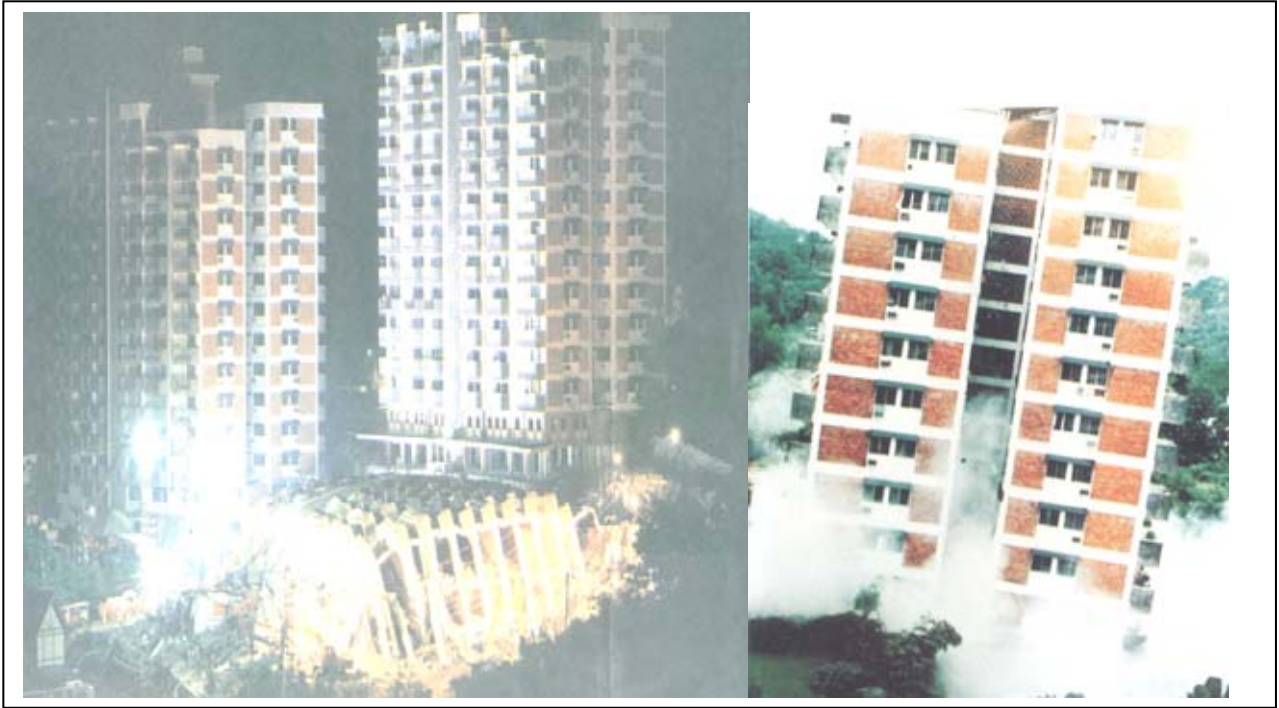
Figure 6: Collapse of Block 1 of the Highland Tower Apartments
