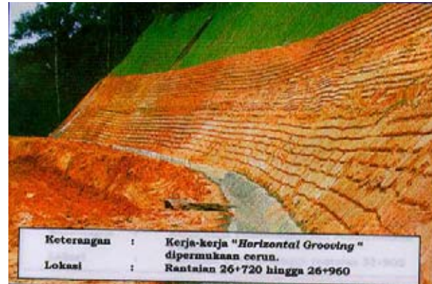
Figure 29: Example of Horizontal Grooves
