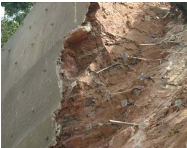
Figure 19: Example of facing failure (after Tan & Chow, 2009)
