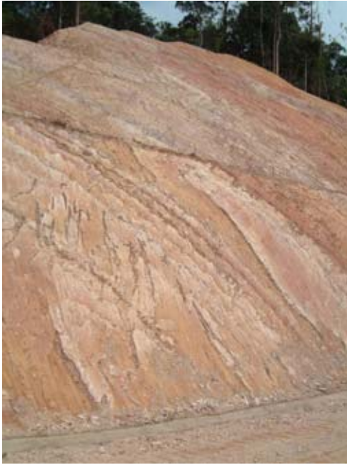
(a) Joints with infilling material
