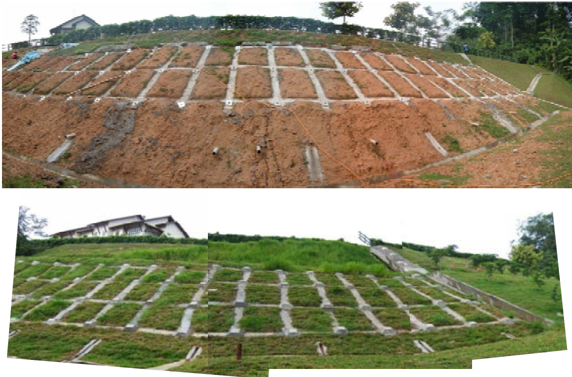
Figure 17: Grid beam system before and after fully grown vegetation (after Liew, 2005a)
