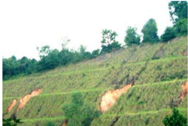
Figure 24: Localized landslips (after Gue & Tan, 2004)
