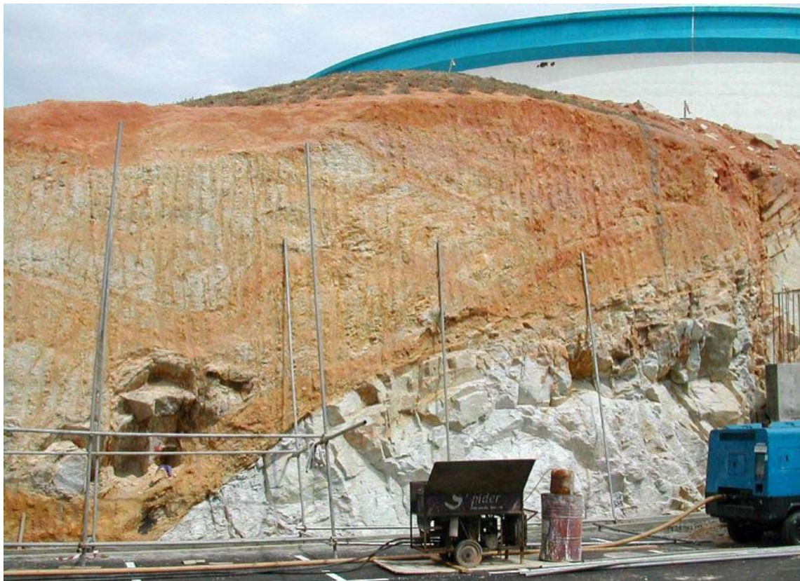
Figure 21: Exposed slope with varying degrees of weathering (after Liew et al, 2004)
