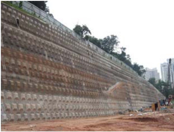
Figure 18: Fully shotcrete soil nail slope in Kuala Lumpur
