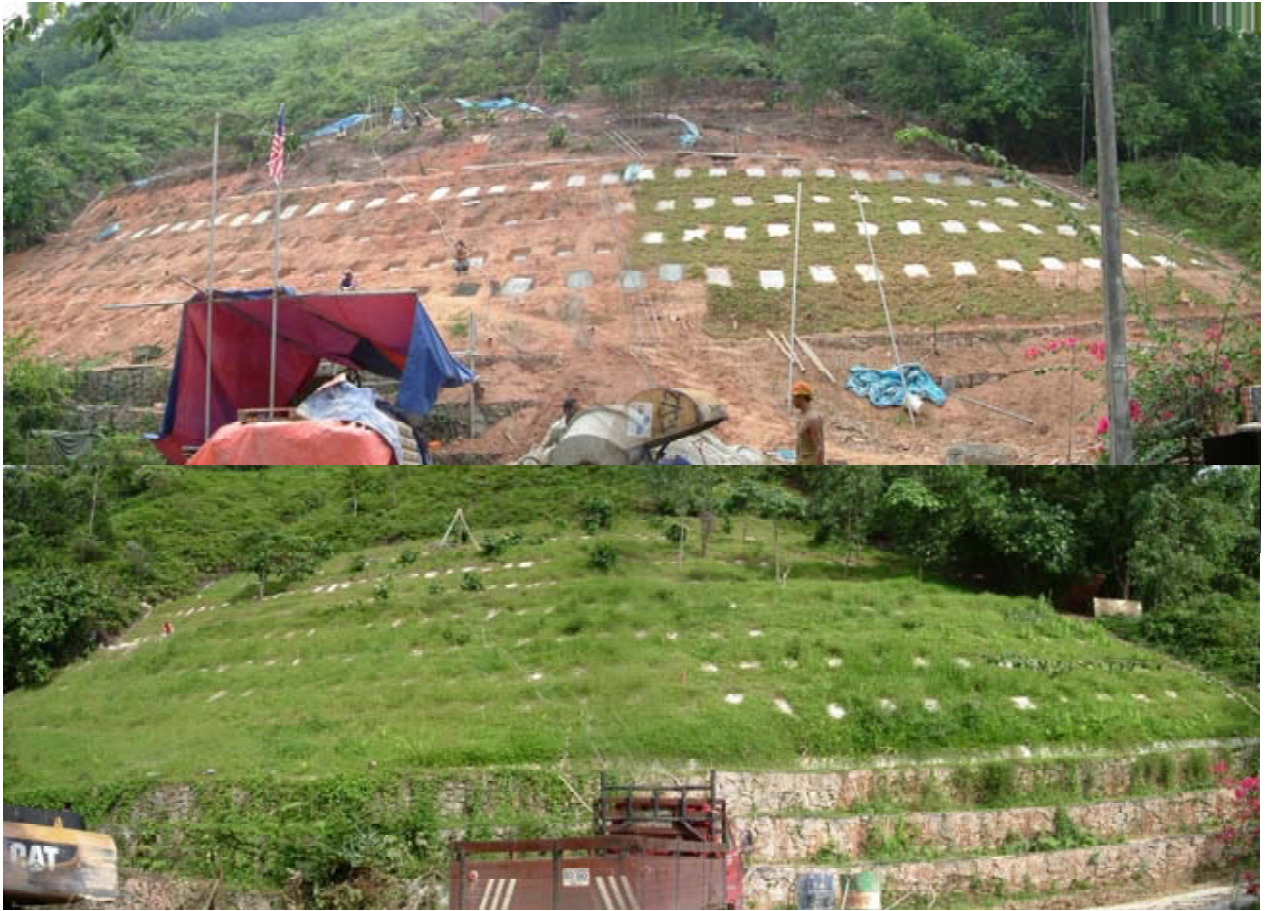
Figure 16: Individual nail head system before and after growth of vegetation (after Liew, 2005a)
