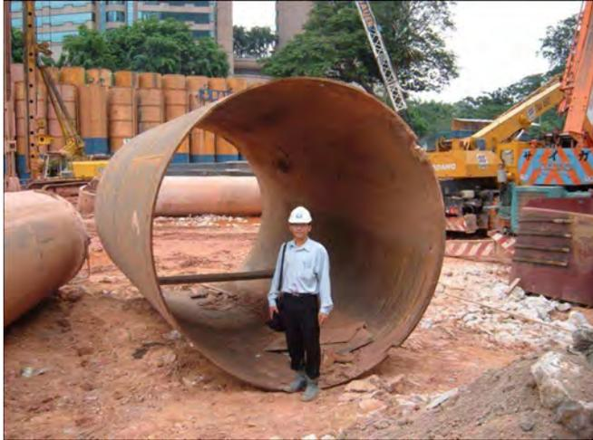
**Fig. 3** Casing for 3.0m diameter bored pile.
