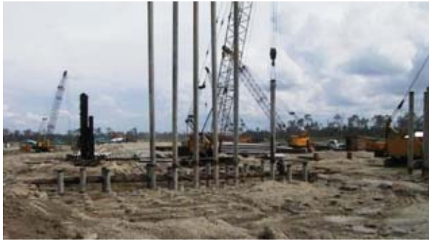
Fig. 12 Installation of Frictional Piled Raft Foundation for Storage Tank
