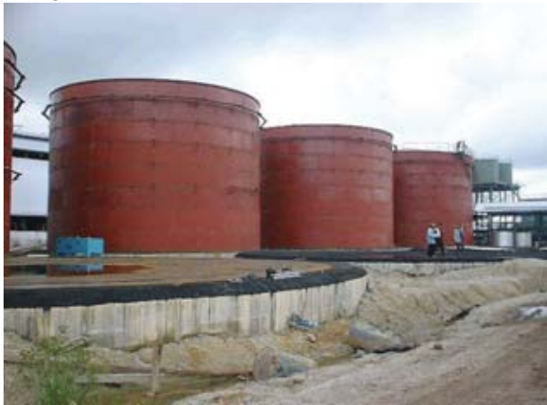
Fig. 13 Completed Storage Tank on Frictional Pile foundation
