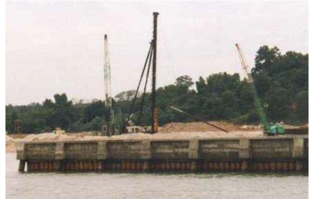
Fig. 17 Completed Structural Breakwater Structure using Pre-stressed Concrete Spun Piles
