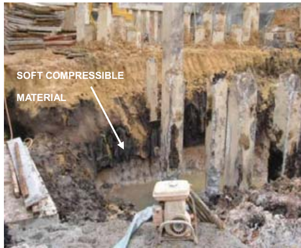
Fig. 16 Soft Compressible Deposit at the Valley as exposed during Pilecap Excavation
