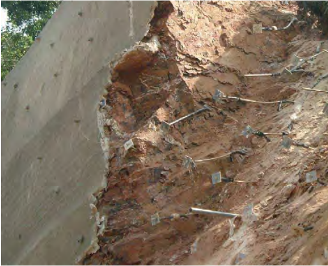
Fig. 10 Example of face failure (side view).
