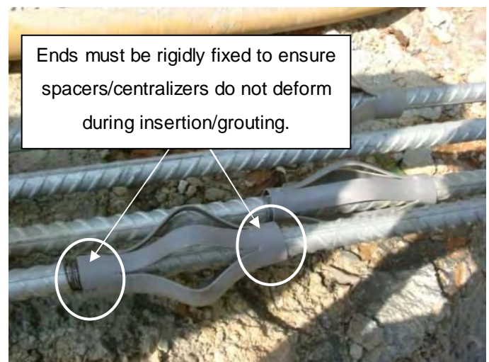
Fig. 7 Typical spacers/centralizers for soil nails.
