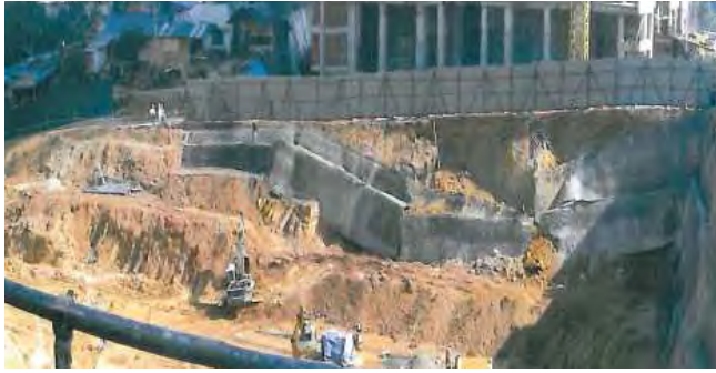
Fig. 16 Failed soil nail slope (Note: Some backfilling works already carried out to stabilize the slope).
