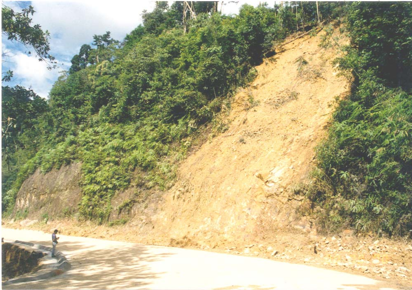
Plate 8 : Landslide L6 on a cut slope which measured about 16 metres high.
