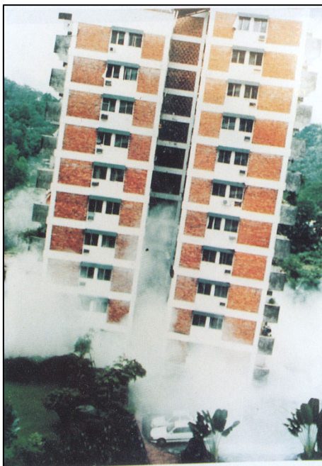
Figure 1. Highland Towers collapse (from MPAJ, 1994)
