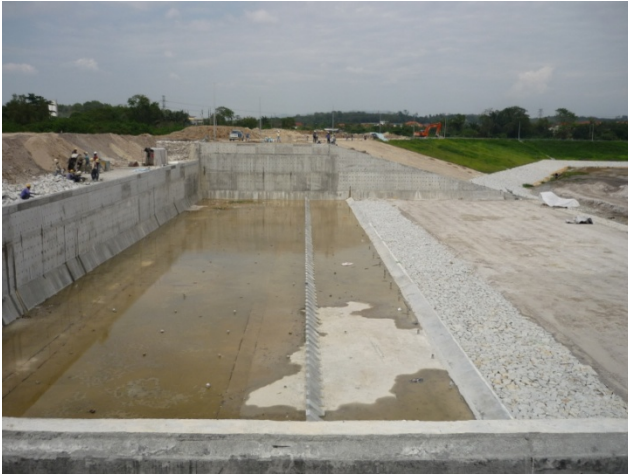
Figure 20. Inlet Structure under Construction.
