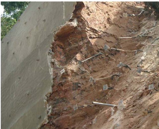
Figure 6. Example of face failure.
