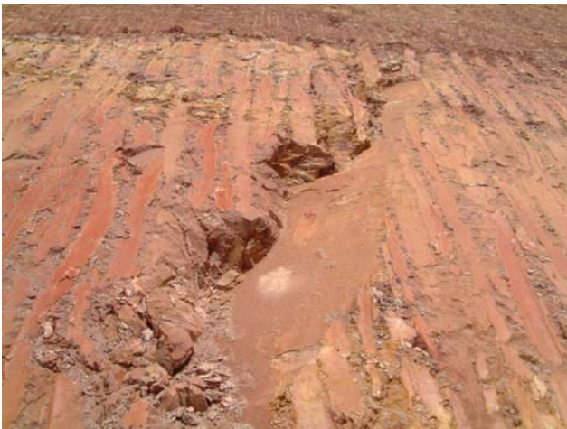
Figure 8. Daylighting joint sets observed on slope.
