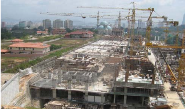
Figure 5. Superstructure works in progress after completion of soil nailing works.
