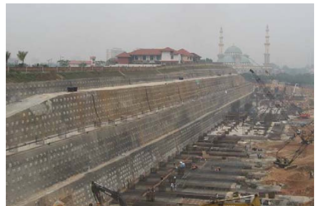
Figure 4. 30m high soil nail slope.
