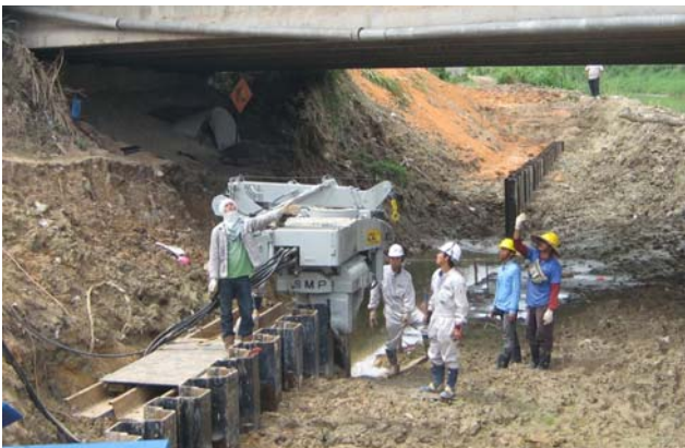
Figure 22. Press-in Sheet Piling Works underneath the Bridge.
