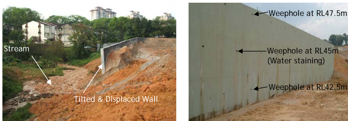
Figure 1: Overall Site Conditions and Water Staining at Weephole Drains
