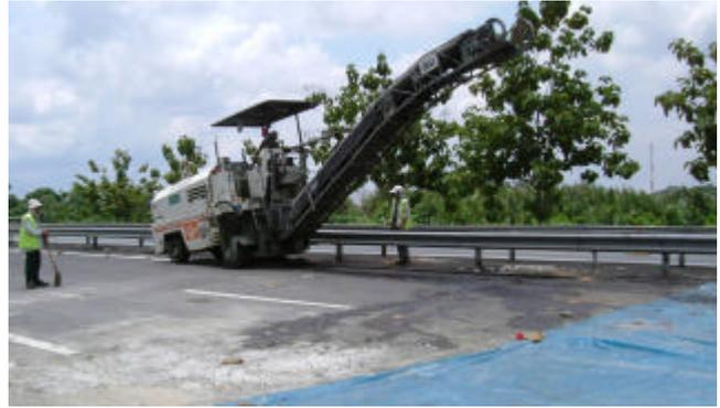
Fig. 11 Milling works in progress
