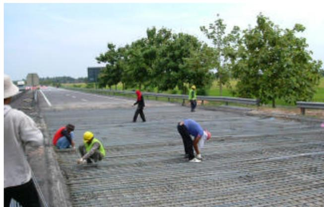
Fig. 13 Laying of steel reinforcement.
