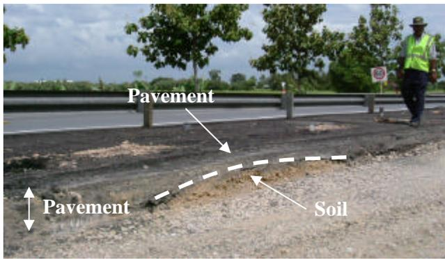
Fig. 3 Differential settlement observed after excavation to depth of about 300mm.
