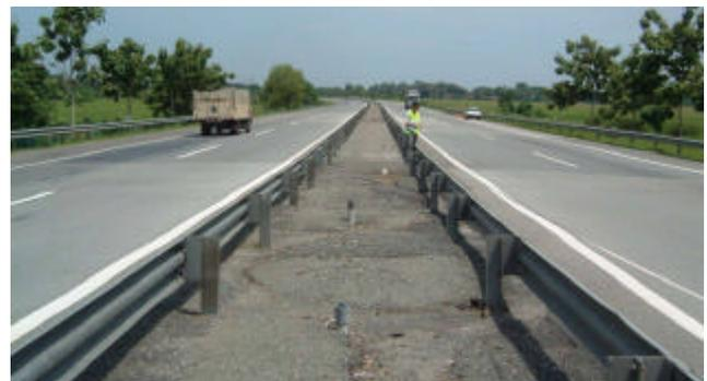
Fig. 1 ‘Mushrooms’ observed at median of expressway. (Note: ‘Mushrooms’ was not observed along carriageway due to regular repaving works)
