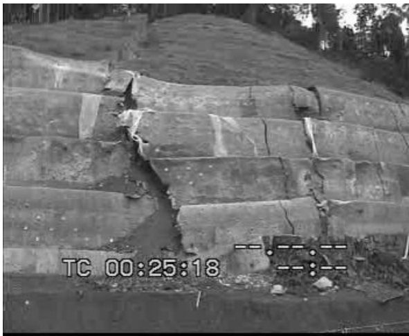
Figure 5. Front view of failed soil nail slope.
