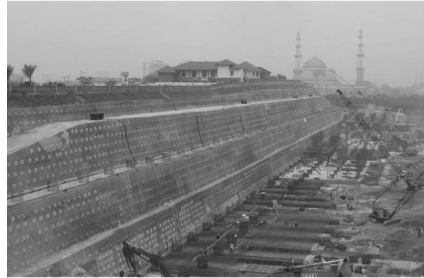
Figure 3. 30m high soil nail slope.
