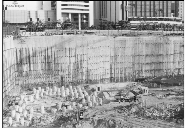
Figure 16. Berjaya Times Square, Kuala Lumpur during construction.
