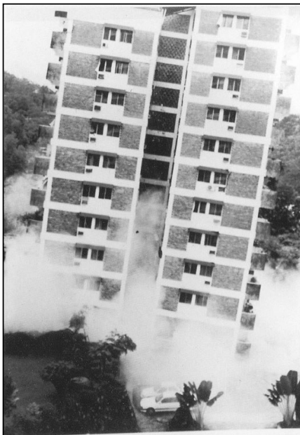
Figure 1 : Block 1 Starts to Topple (from MPAJ, 1994)
