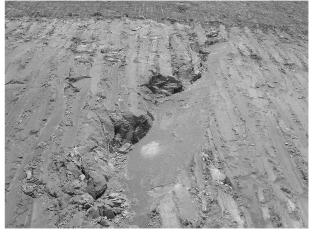
Figure 6. Daylighting joint sets observed on slope.
