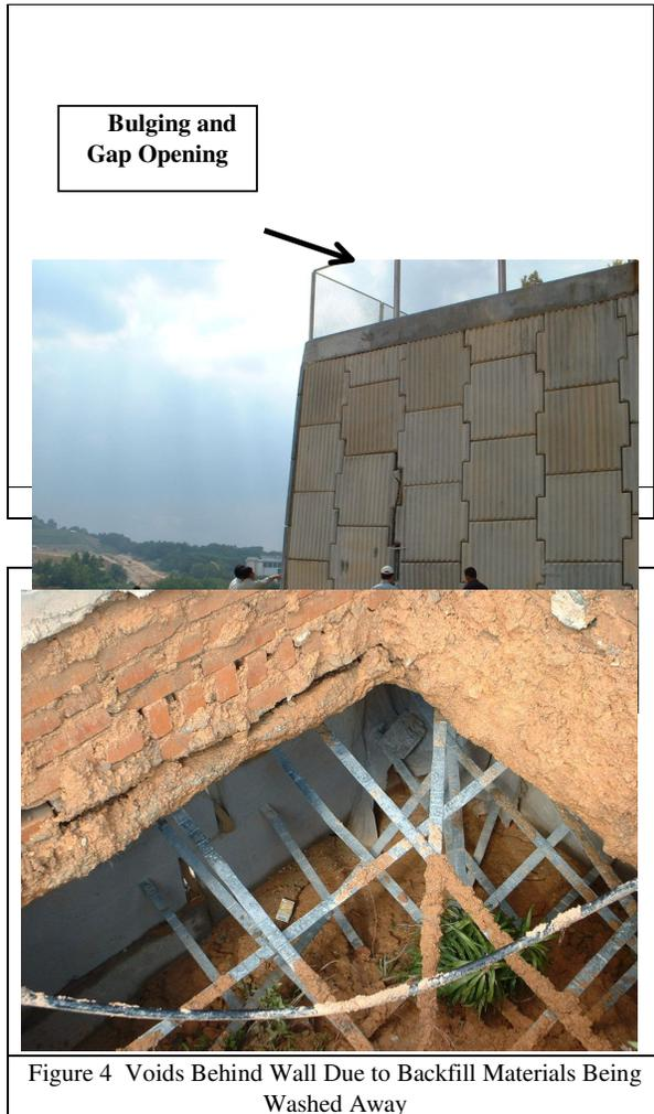
Figure 4 Voids Behind Wall Due to Backfill Materials Being Washed Away
