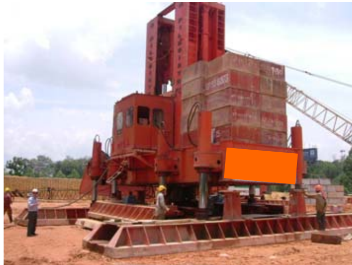
Figure 7: Typical hydraulic jack-in piling system used in Malaysia
