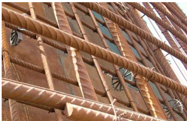
Figure 6: Plastic reinforcement spacers
