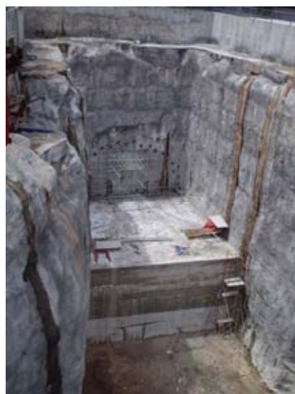
Figure 15: Foamed concrete application at the SMART tunnel in Kuala Lumpur (after Lee & Yung, 2005)
