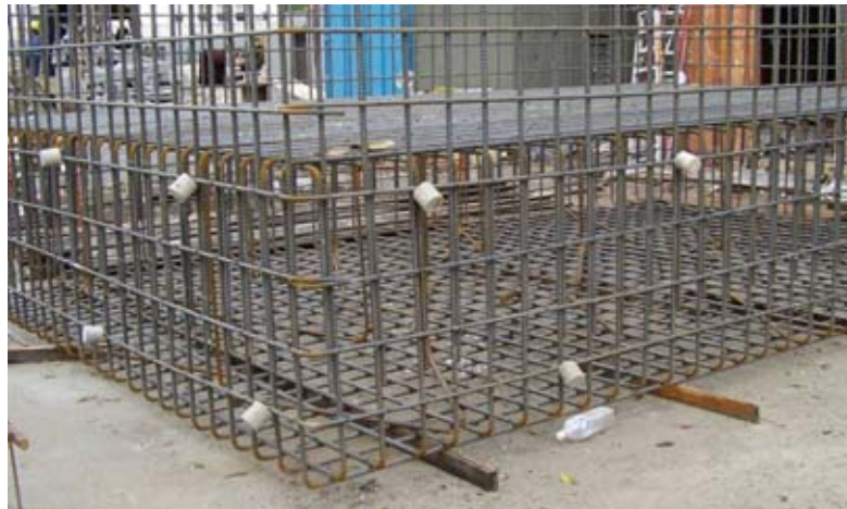
Figure 5: Cast at-site reinforcement spacers
