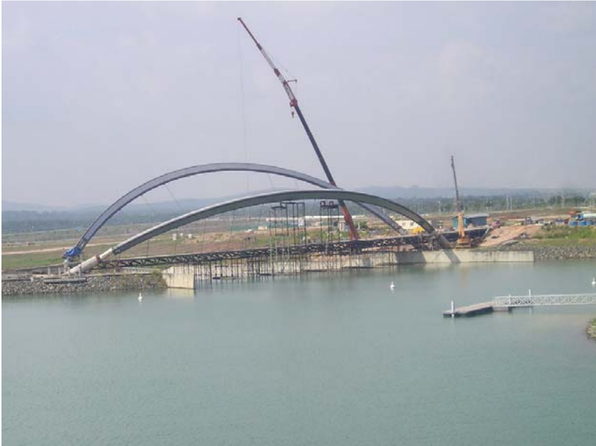
Figure 9: Bridge construction using IBS system ( http://www.eng.upm.edu.my/hrc/fotogaleri/BHS2004/visit/pic33v.jpg )
