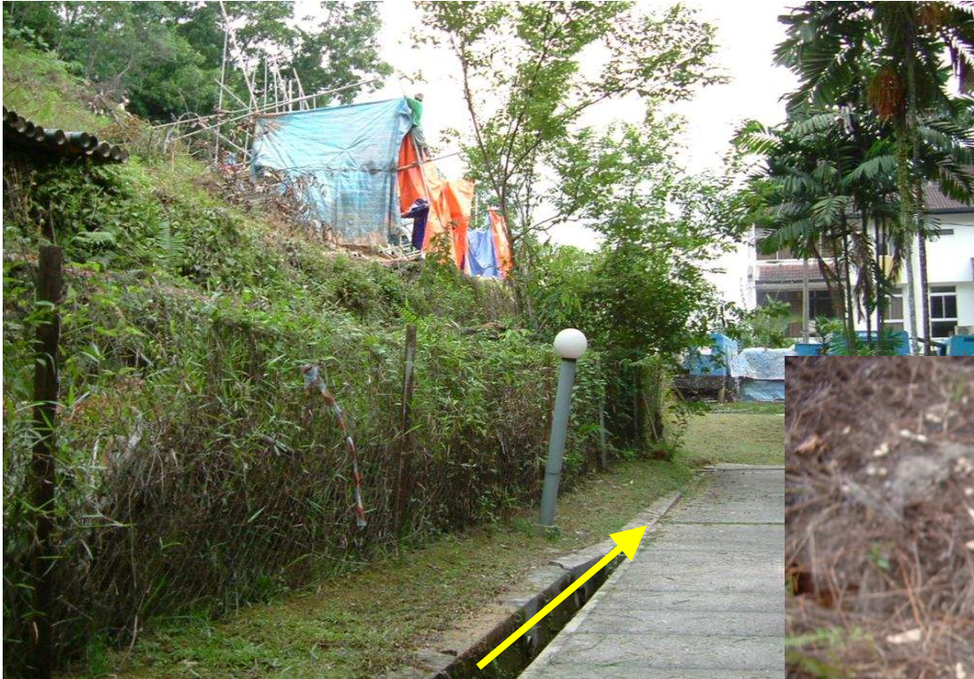
Closed Drain at Toe of Slope
