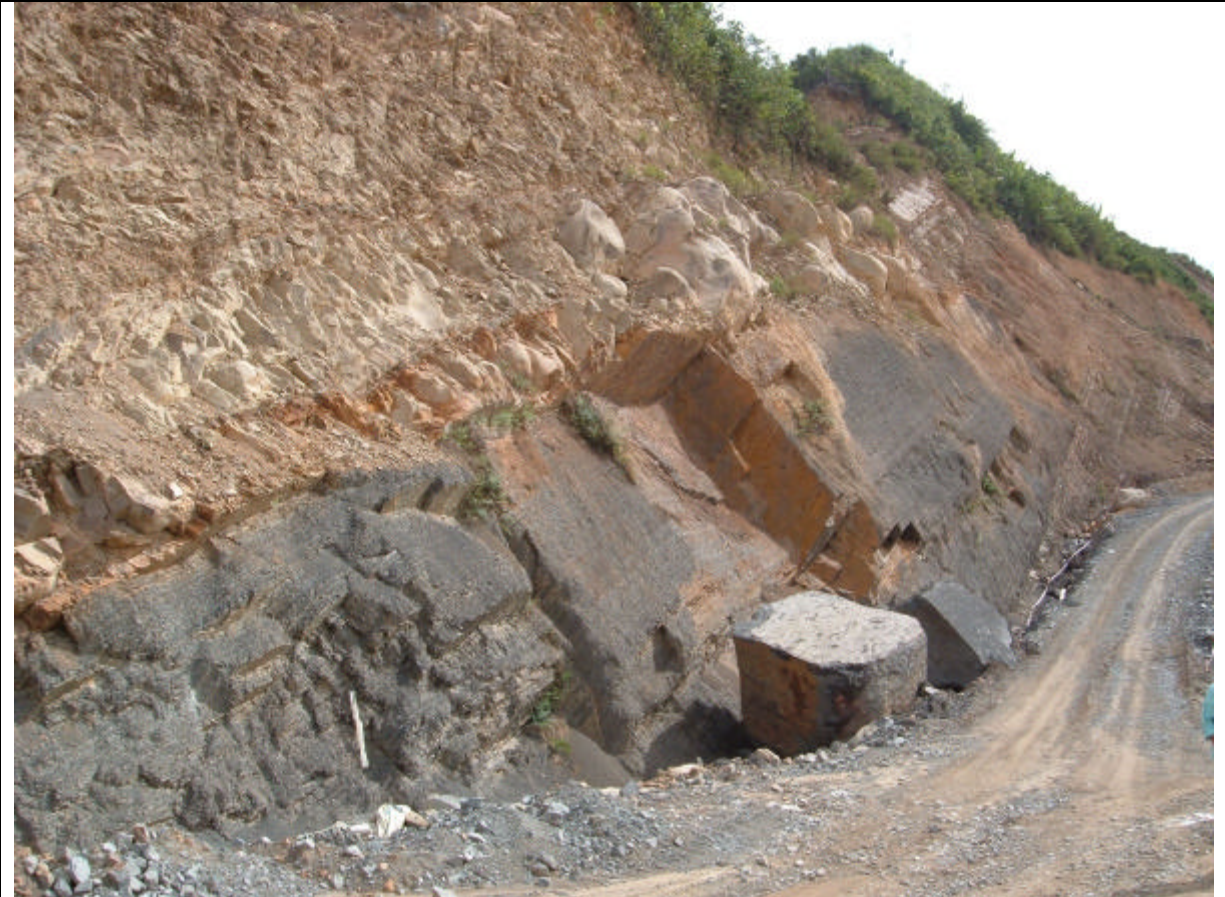
Figure 8 : Block Failure of Sedimentary Formation
