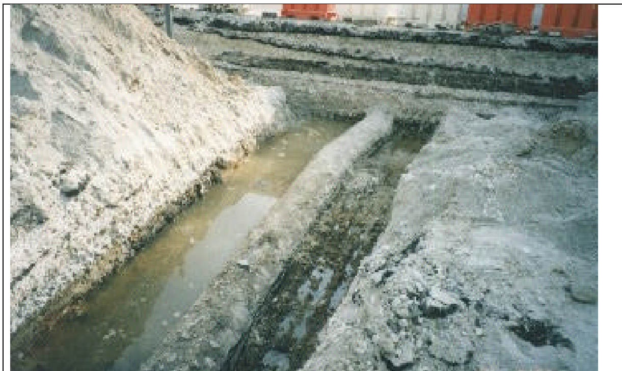
Figure 14 : Water Carrying Services running across the proposed Highway Alignment
