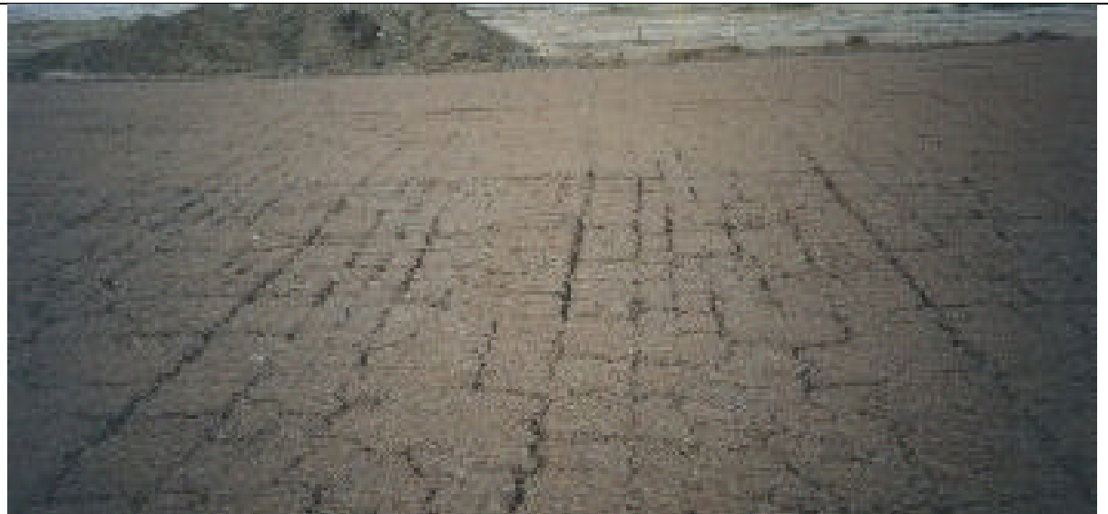
Figure 12 Shrinkage Cracks at Runway Subgrade
