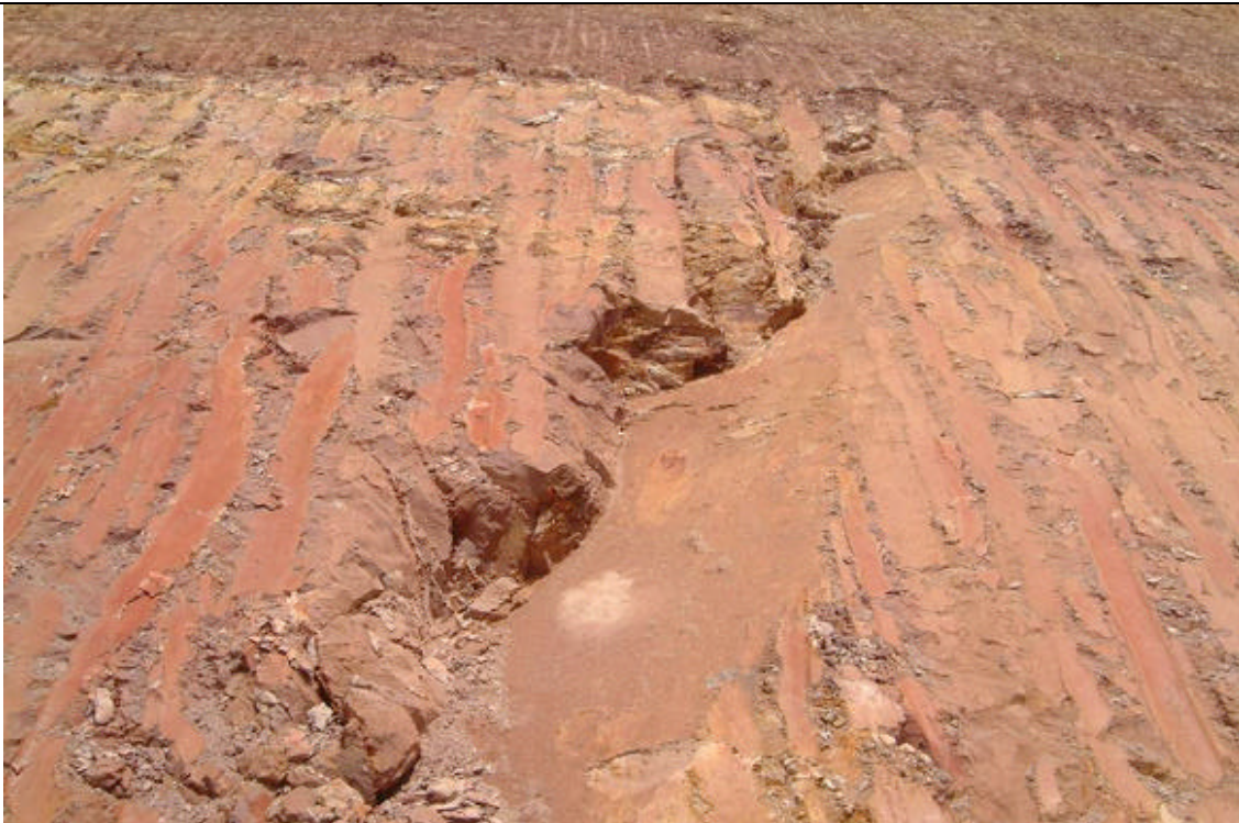
Figure 3 : Localised Wedge Failure contributed from Day-lighting Joint Sets and Beddings of Cut Slope Towards Road Alignment
