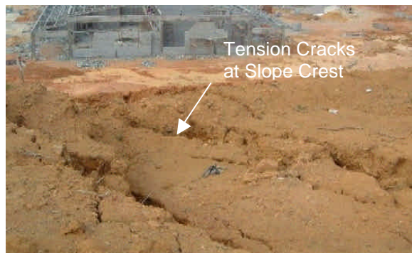
Figure 3 Tension Cracks at Top of Slope
