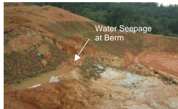
Figure 4 Water Seepage at Berm
