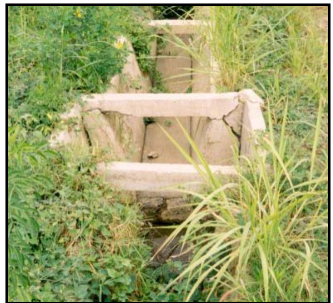
Photo 6: Distorted Drain Sump
