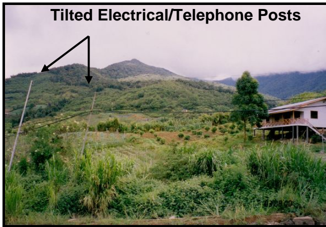
Photo 2: Tilted Electrical/Telephone Posts
