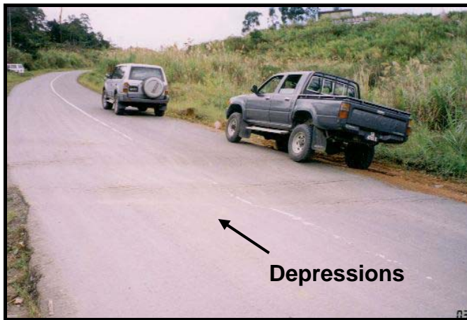
Photo 8: Depression on Road Pavement
