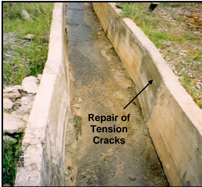
Photo 7: Repaired Cracked Drain
