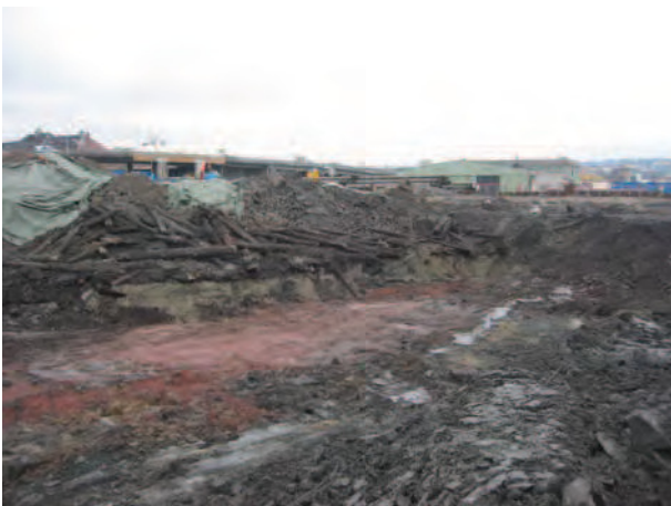
Excavation of contaminated ground before remediation
