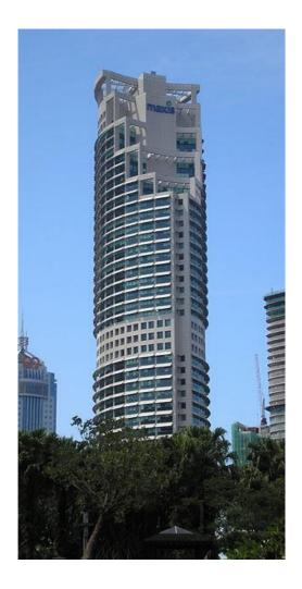
During the employment with Ranhill, Ir. NG had led a team of structural engineers to design and supervision of the 60-storey Maxis Tower at the heart of Kuala Lumpur City Center. It was one of the first office building in Malaysia to adopt Post-tensioned banded beams system. The usage of prestressed concrete had proven more efficient in term of time and cost.
