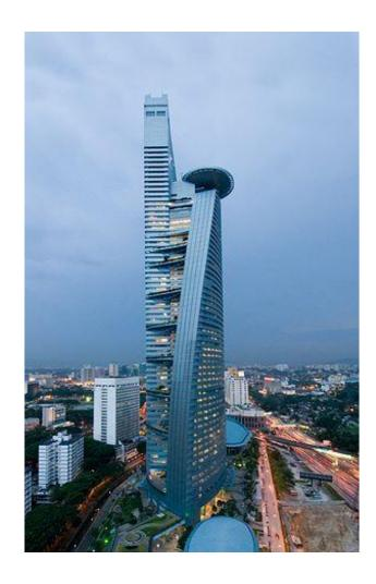
During the employment with Ranhill, Ir. NG had led a team of structural engineers to design and supervision of the 310m Telekom Tower at the heart of Kuala Lumpur City Center. It was Post-tensioned banded beams system, with special design with taper beam-column interface to accommodate the M&E services passage. The usage of prestressed concrete had proven more efficient in term of time and cost.
