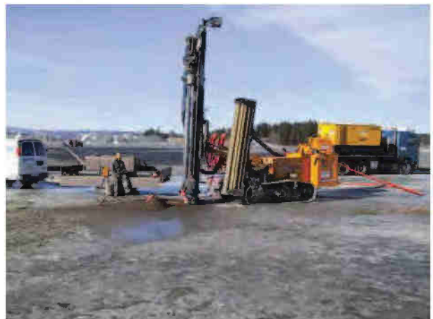
Installation of groundwater wells for environmental site assessment
