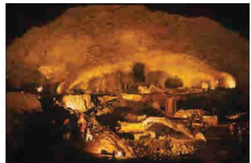
The Olympic rock cavern in Gjøvik, Norway, with 62 m span and 91 m length, is the world's largest rock cavern for public use.
