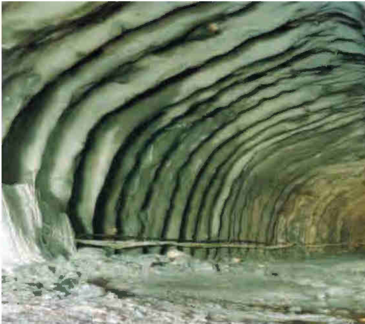
New 22 m span metro station in downtown Oslo constructed with cover of only 3-5 m of poor quality rock; reinforced shotcrete ribs were used for temporary and permanent support.
