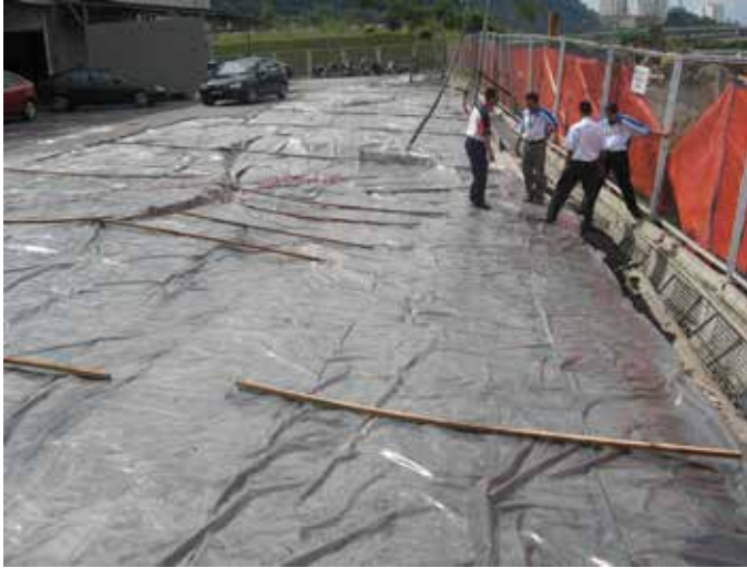
Ground Distress at Active Wedge
