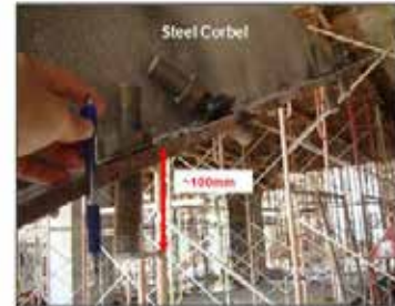
Post-installed Bolts After Wall Failure
