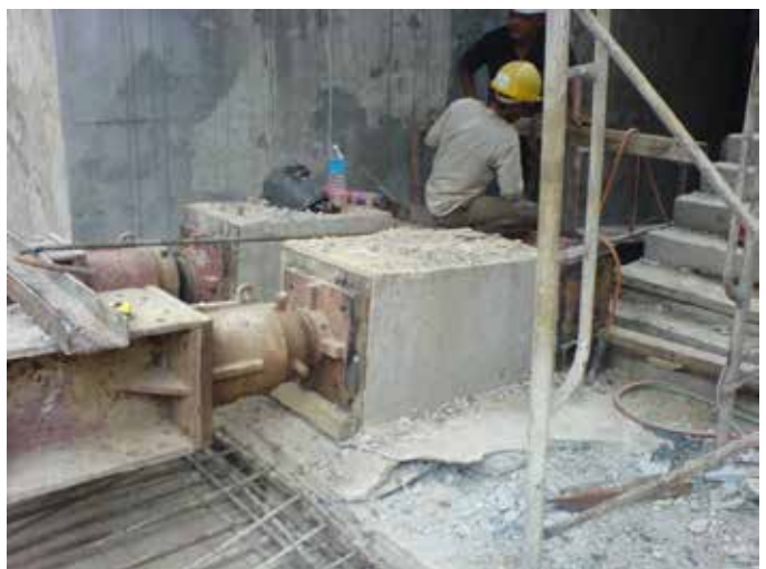
Shear Failure of Corbel Support
