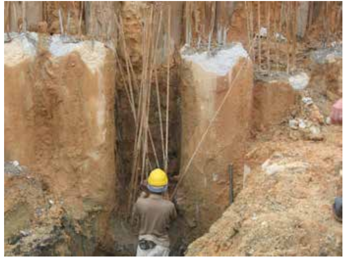
Repairing of CBP Pile
