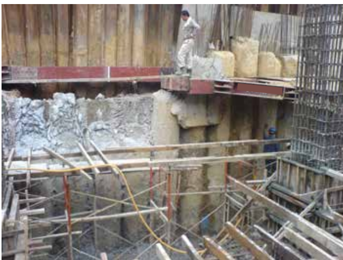
Repairing Crushed CBP
