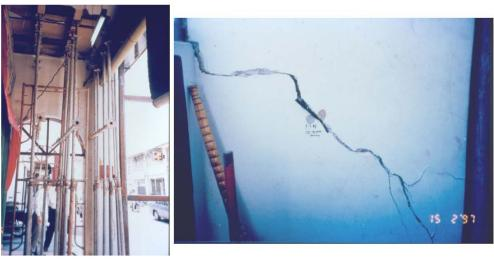
Deep excavation in Alluvium with sand layer lowered the water table to a distance of over 40 times the depth of excavation & induced settlements up to 120m away from excavation!
