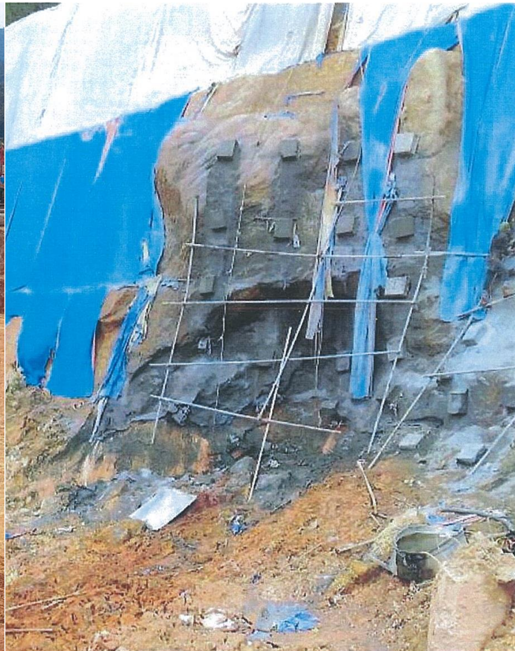
Instability During Soil Nail Installation 5th May 2017- (2nd Slip)
