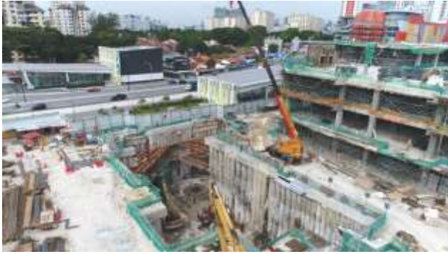
Fig. 7. Overview of Excavation Works
