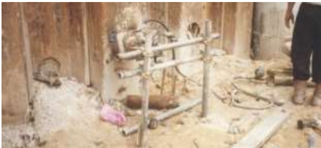
Fig. 12. View of the Pull-Out Test Arrangement
