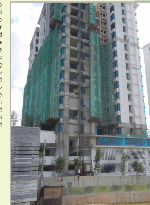
• 20 Floors Jadite Suites Under Construction
