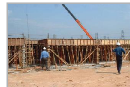
• Erection of Superstructure
