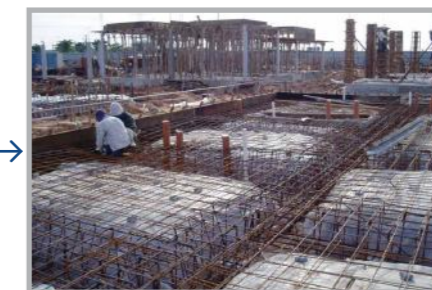
• Laying of Reinforcement Bars
