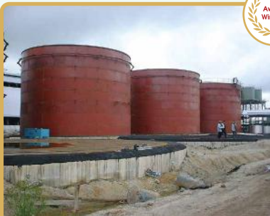
Indonesia Pulau Palm Oil Mill
