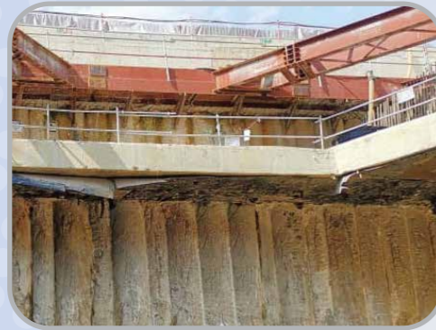
Secant Bored Pile Wall
