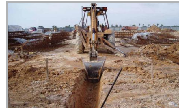
• Strip-footing Excavation
