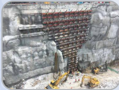
Support System • Ground Anchor
