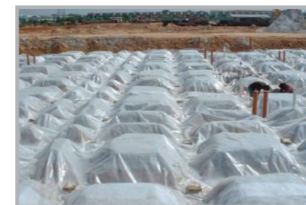
• Laying of Plastic Sheet Lining
