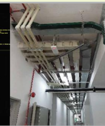
• Installation on Site
