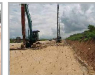
Typical PVD Machine working beside the Live Track
