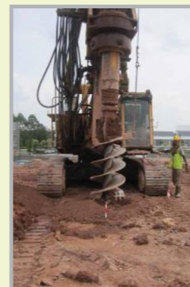
• Rotary Auger Bored Piling
