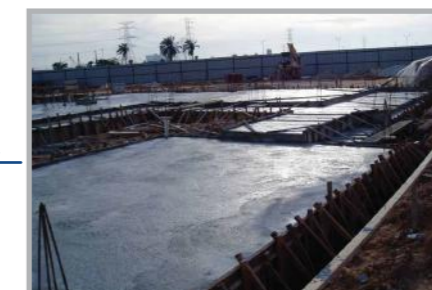
• Casting of Strip-raft Foundation
