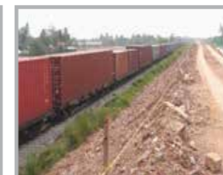
Embankment fill with surcharge next to existing live tracks
