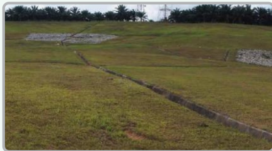
Slope Remedial works at North-South Expressway
