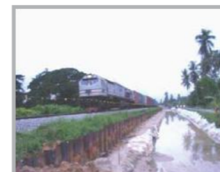
Temporary Sheet Pile for Excavation and Replace Method (E&R).
