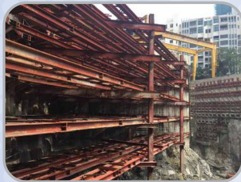
Support System • Steel Strutting
