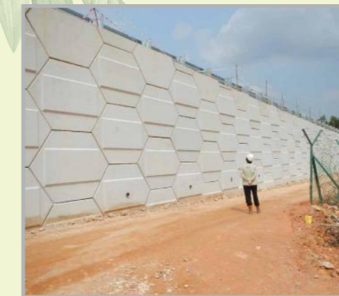
• Reinforced Soil Retaining Wall
