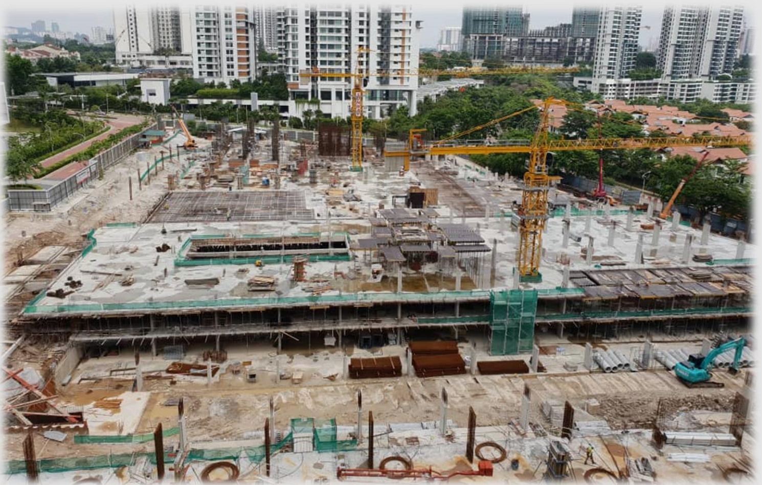
Figure1: Overall Site Progress of RC1
