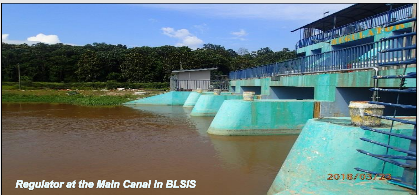
Bernam River Headwork diverts water to BLSIS
