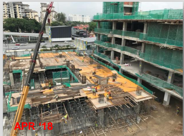
Construction of Above-Ground Structure
