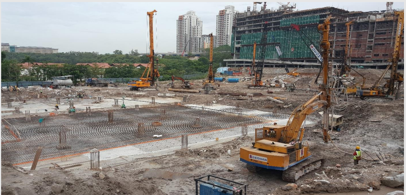
Completion of Sub-structure Works
