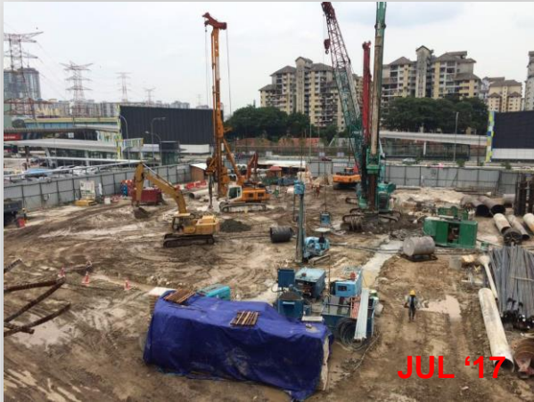
Construction of Contiguous Bored Pile Wall
