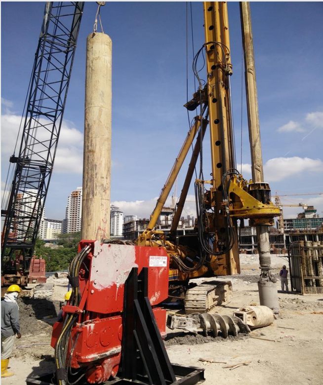
Bored Piling Works
