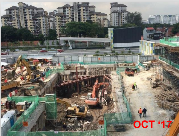
Installation of Temporary Strut
