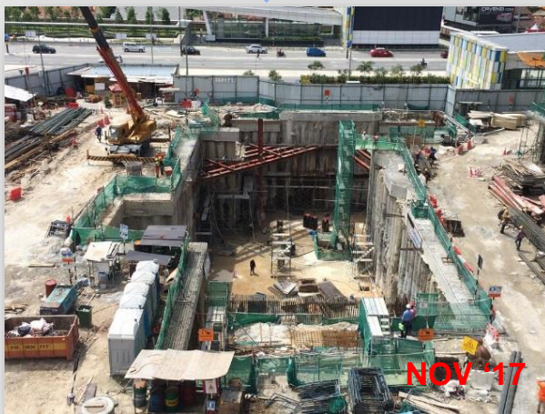
Excavation to Final Excavation Level
