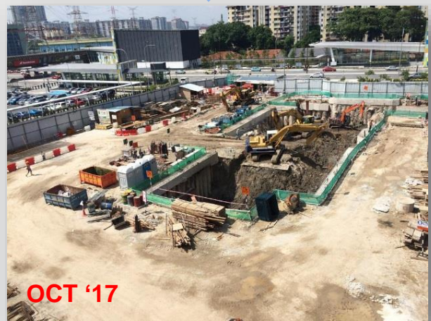
Excavation Works in progress
