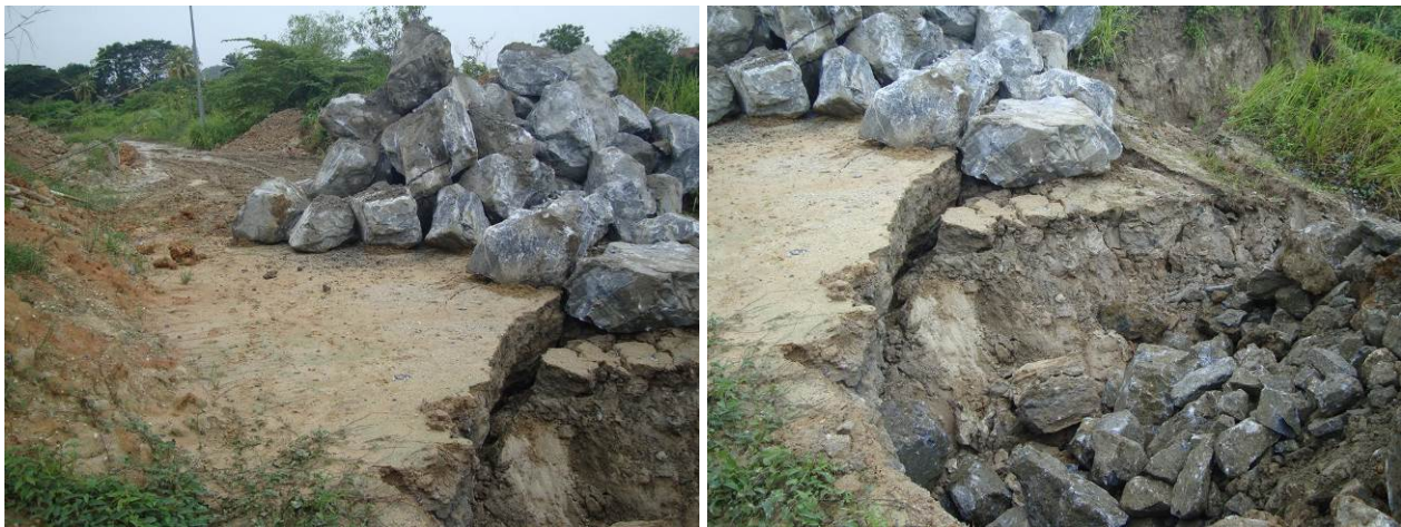
Plate 12: Sequential dumping rock fragments of varying sizes to infill the solution channel for plugging
