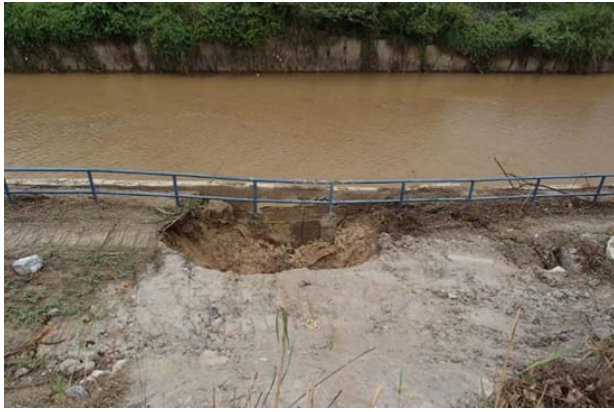
Plate 9: Sinkhole developed behind channelised river section with solution channel connection to quarry benches
