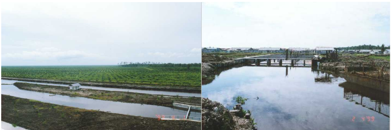
Plate 4: General view of irrigation drainage and transportation network with overflow weir structure at canal system regulating water level at the oil palm plantation estate
