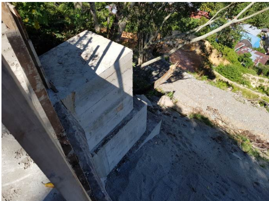
Plate 21: Reinforced concrete buttress abutting to huge diorite boulder
