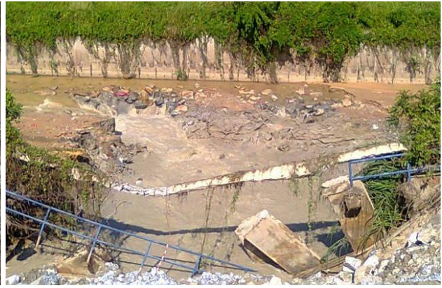
Plate 9: Sinkhole developed behind channelised river section with solution channel connection to quarry benches
