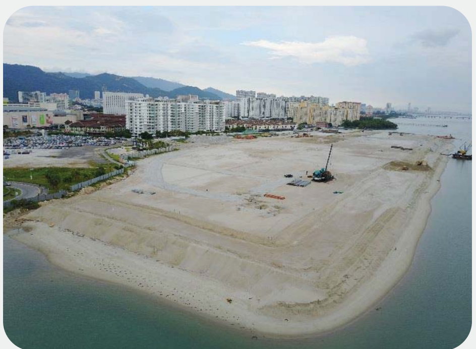
Figure 2: Site Photo: On-going Land Reclamation Works
