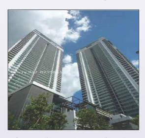
10 @Mont Kiara, 2 blocks of 45-storey condominium towers using jack-in spun piles with sizes ranging from Ø400mm to Ø600mm.
