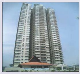
Mont' Kiara Banyan, 1 blocks of 32storey condominium towers using jack-in spun piles with sizes ranging from Ø300mm to Ø450mm.
