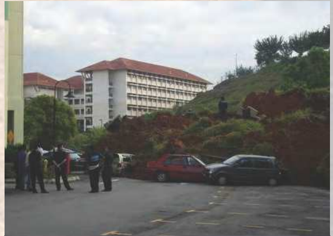
Slope failure at Precinct 9, Putrajaya
