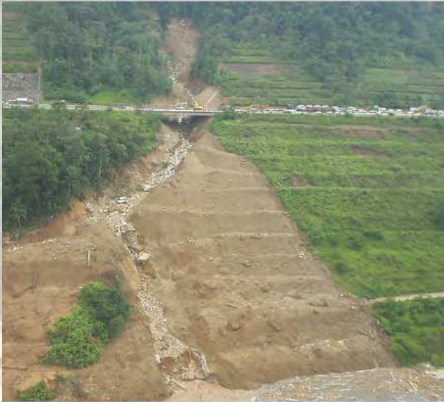
Debris flow at KM302 of PLUS Expressway
