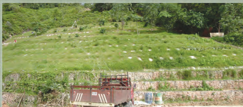
Figure 6: Green Pad Facing (After Closed Turfing)
