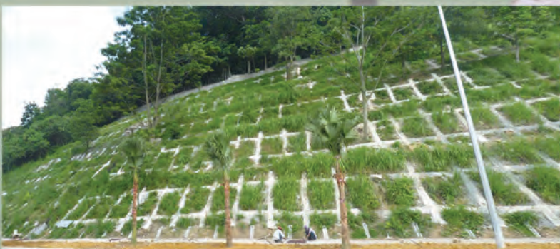
Figure 3: Grid Beam Facing Upon Completion (With spot turfing)
