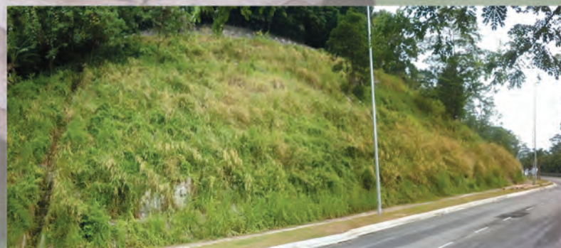
Figure 4: Grid Beam Facing (With fully grown spot turfing)
