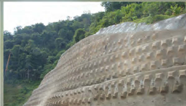
Figure 1: Typical Shotcrete Facing (Before Planting of Creepers)
