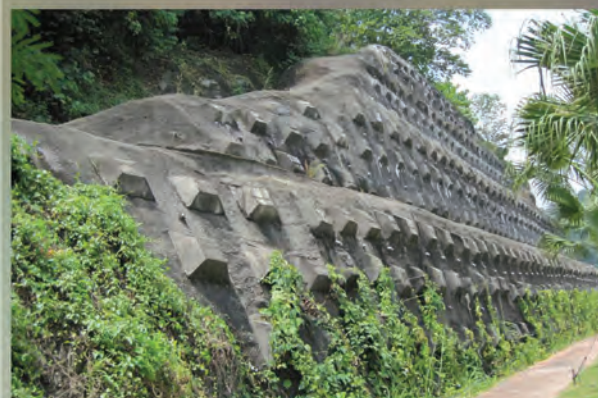
Figure 2: Typical Shotcrete Facing (After Planting of Creepers)
