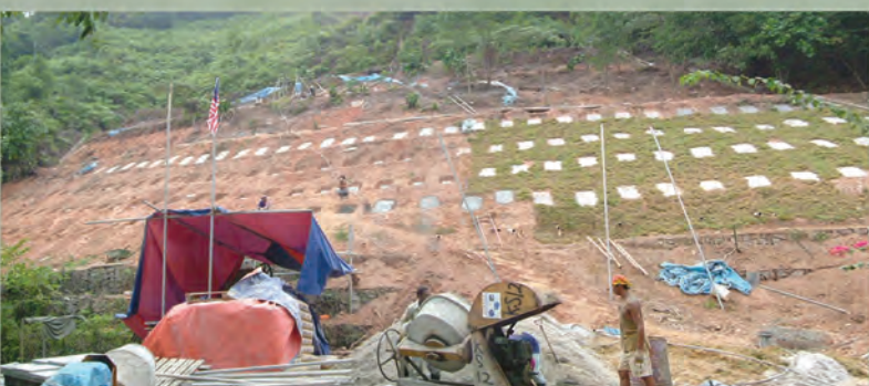
Figure 5: Pad Facing During Construction (Before Closed Turfing)
