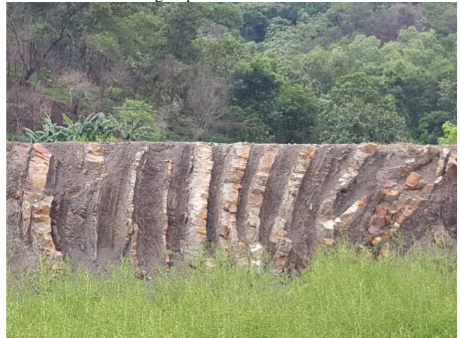
Figure 1 Exposed Rock Slope with Sub-vertical Bedding
