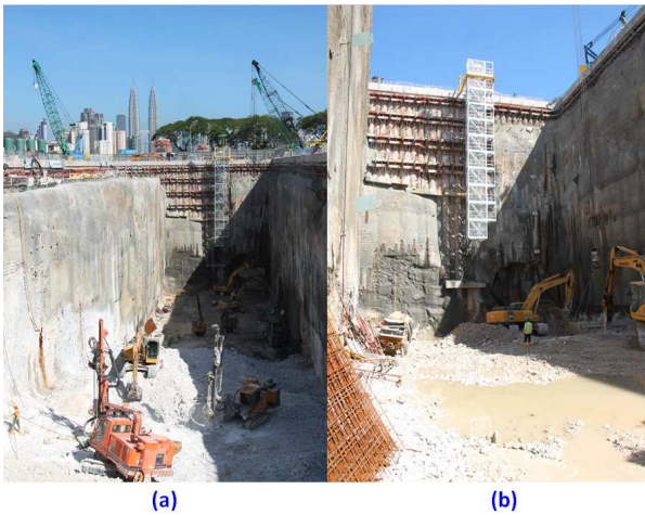
Figure 5. Overall view of excavation works
