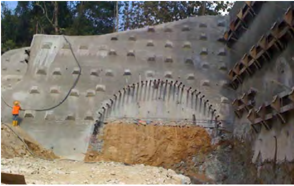
Fig. 4. Soil nailed wall for tunnel face
