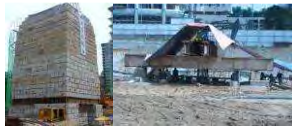
Fig. 1 4560 Tons Maintained Static Pile Load Test & 1120 Tons Tension Pile Load Test
