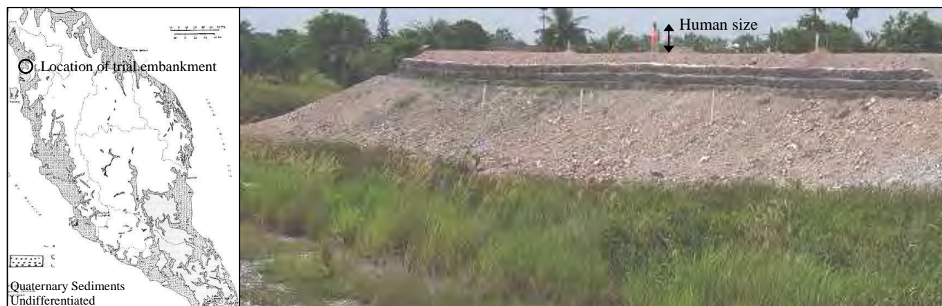
Figure 1 Location and overview of instrumented trial embankment
