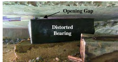
Figure 9 Shearing distortion of rubber bearing
