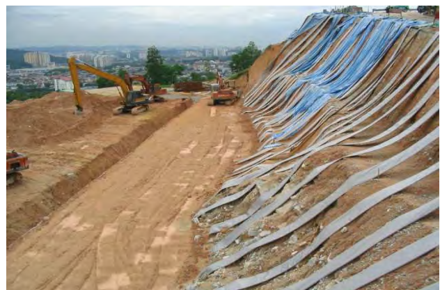
Figure 10 Laying of Strip Drain
