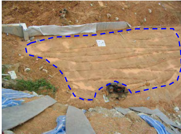
Figure 11 Wet Backfill Material
