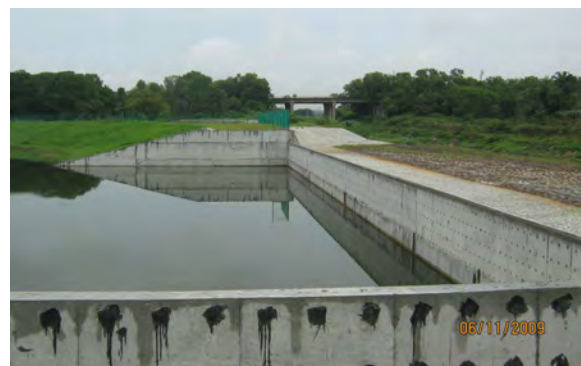
Figure 2 View of the SAS Inlet Structure
