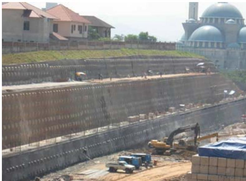
Fig. 28. View of soil nail wall during construction (photo taken in 2006).
