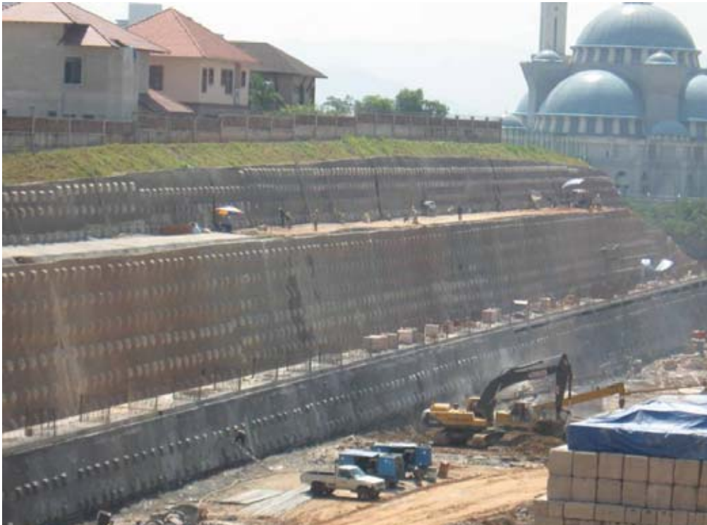
Figure 21: 30m high soil nailed slope in construction in Kuala Lumpur.
