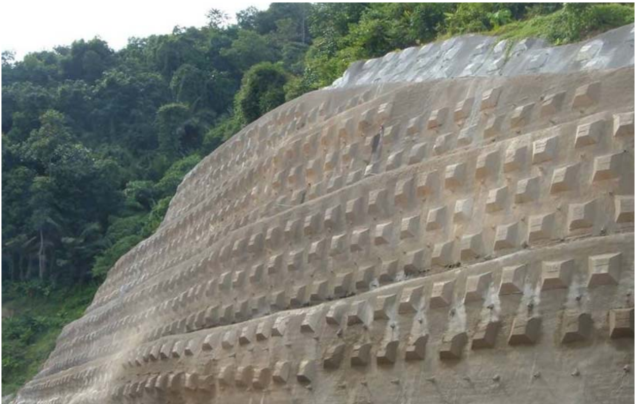
Figure 20: 20m high soil nailed slope in Kuala Lumpur.
