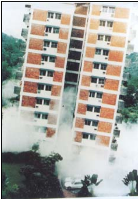
Figure 1 : Block 1 Starts to Topple (from MPAJ, 1994)
