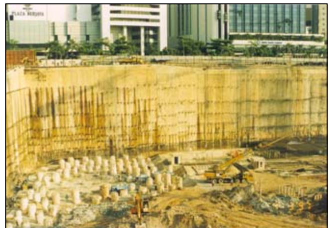
Figure 7. Berjaya Times Square, Kuala Lumpur during construction.
