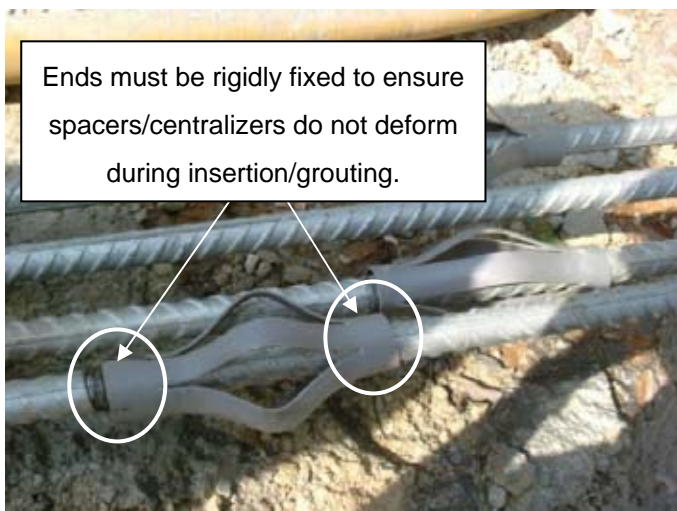
Figure 3. Typical spacers/centralizers for soil nails.
