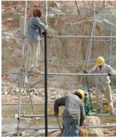
Figure 5: Vertical Grouting of Corrugated Pipe
