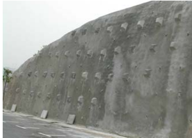
Figure 10: Completed Soil Nailed Slope
