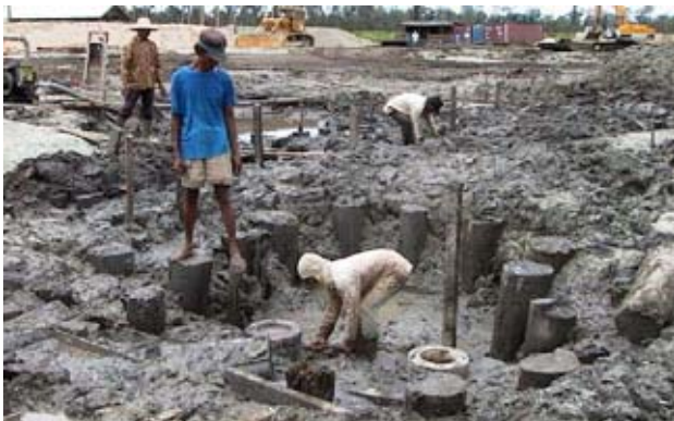
Figure 6 Floating Piles for Structures
