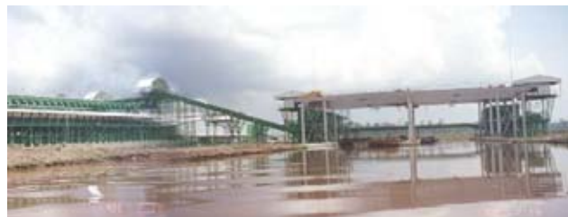
Figure 13 Overview of FFB Crane Bay Design Feedbacks from Instrumentation Results
