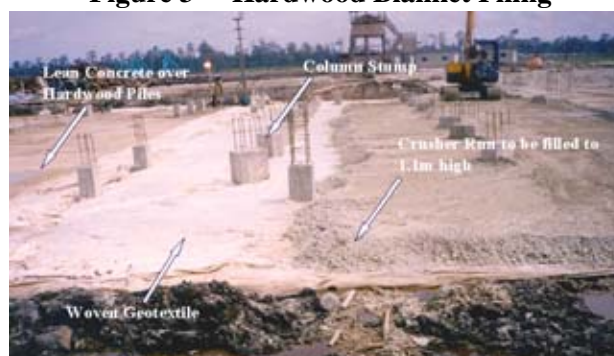
Figure 4 Hardwood Piled Foundations for Platform & Structures
