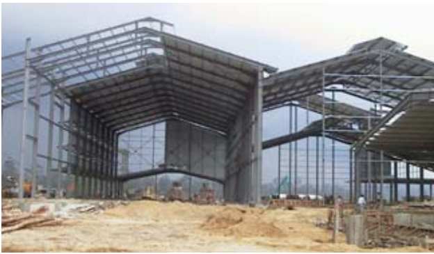
Figure 5 Partially Completed Mill Structure
