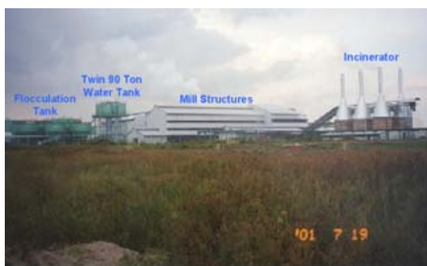
Figure 15 Overview of Completed Mill Structures
