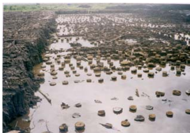
Figure 3 Hardwood Blanket Piling
