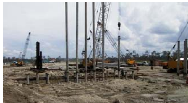
Figure 8 Piled Raft Foundation for Storage Tank
