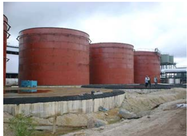
Figure 7 Completed Tank Structures
