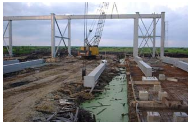
Figure 12 Erection of Steel Frame of FFB Crane Bay
