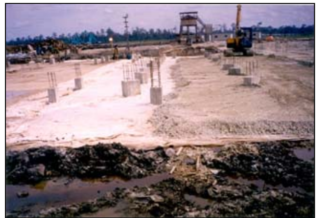
Figure 12 : Hardwood Piled Foundations for Platform & Structures
