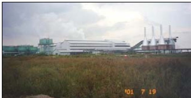
Figure 21 : Overview of Completed Mill Structures
