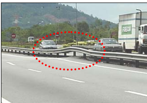
Figure 1 : Hump over piled culvert
