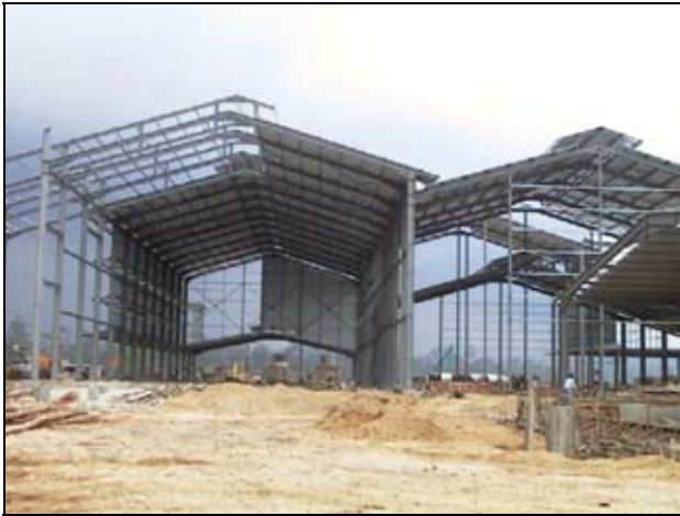
Figure 13 : Partially Completed Mill Structure
