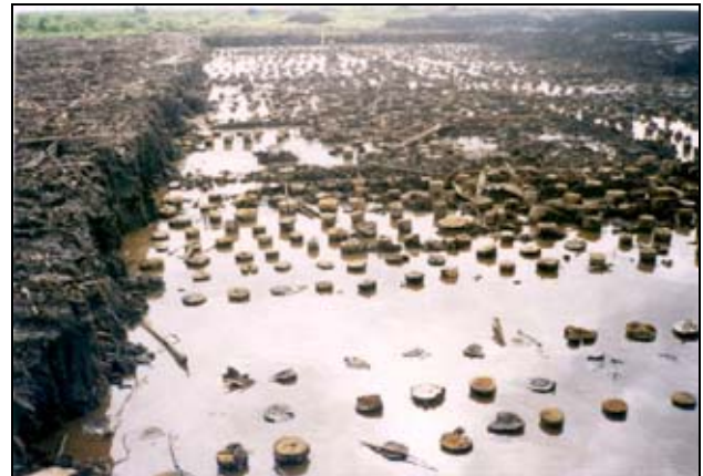
Figure 11 : Hardwood Blanket Piling
