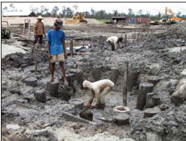
Figure 14 : Floating Piles for Structures
