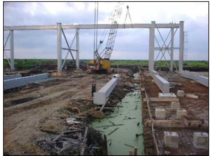
Figure 19 Erection of Steel Frame of FFB Crane Bay
