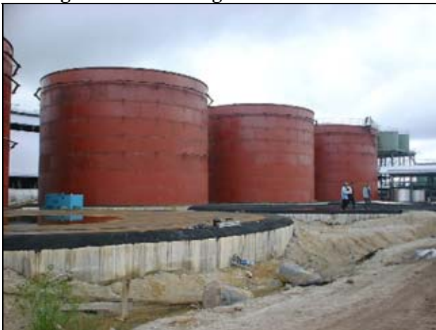
Figure 15 : Completed Tank Structures
