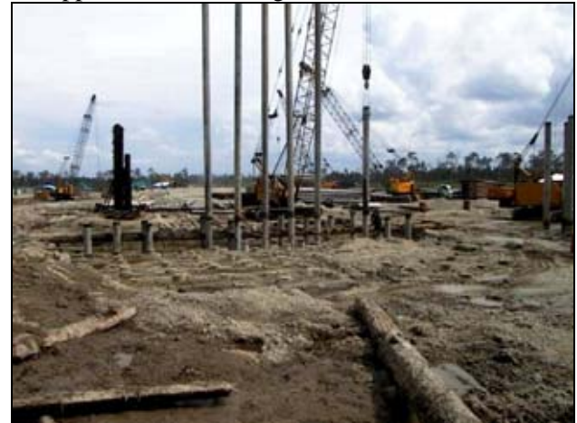
Figure 16 : Piled Raft Foundation for Storage Tank
