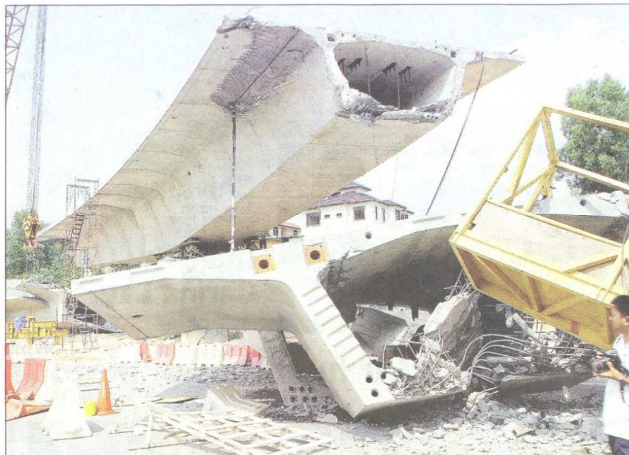
MANGLED WRECK: A section of the collapsed flyover and the gondola of the NKVE-Jalan Meru Link flyover
