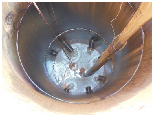
Figure 9 A total of 3 pumping wells were installed at site
