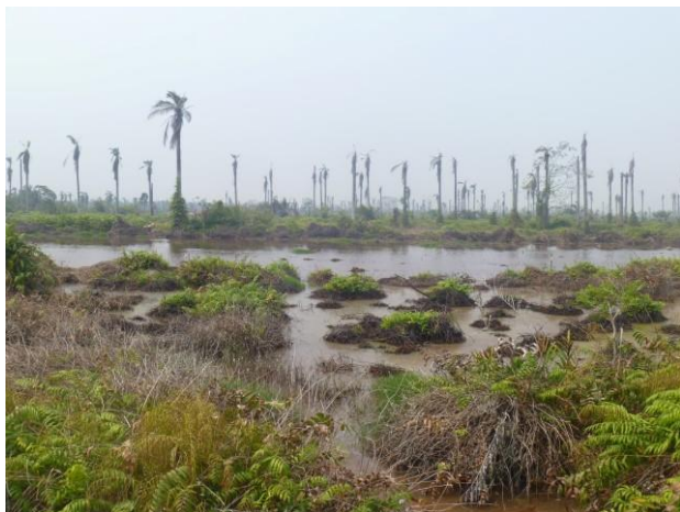
Figure 2. Existing ground condition before site clearing.
