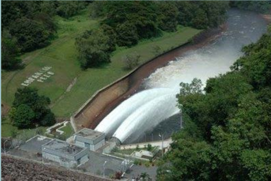
Irrigation Dam – Pedu Dam ( Alor Setar )
