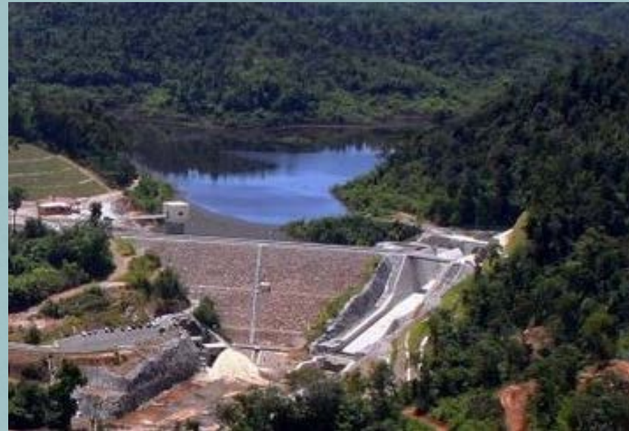
Flood Defense Dam – Beris Dam ( Kedah )
