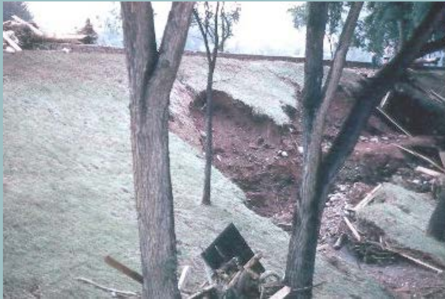
Erosion at the Downstream Face of Dam
