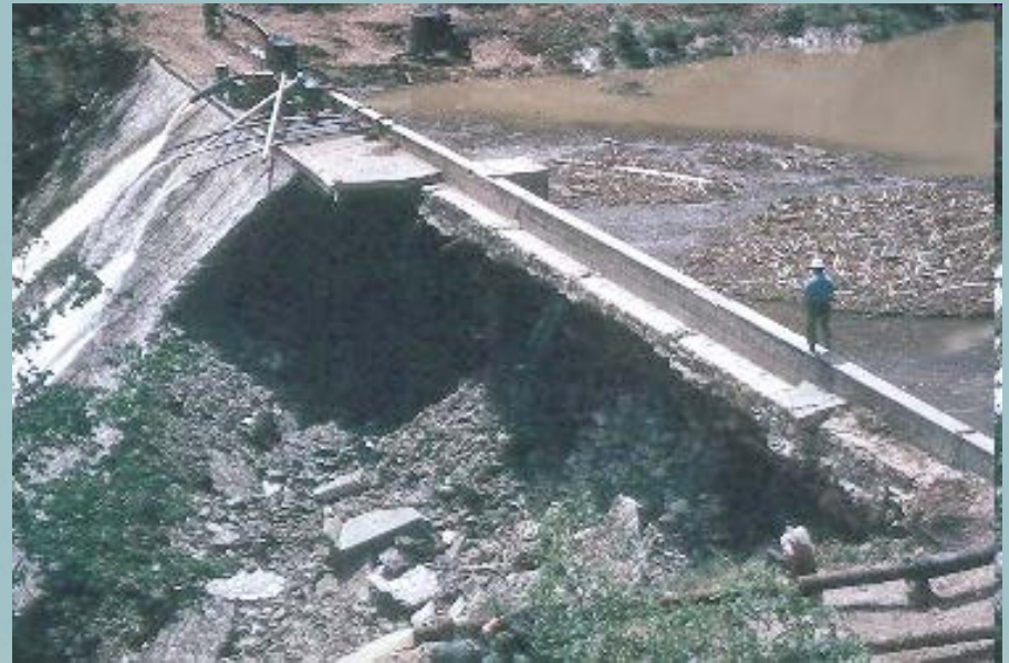
Erosion due to Dam Overtopped
