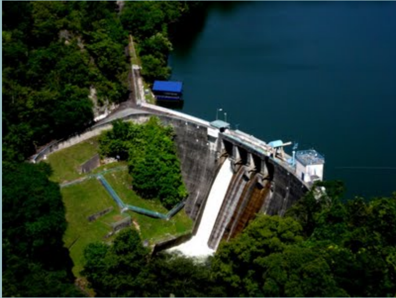
Water Supply Dam – Klang Gates ( Taman Melawati )
