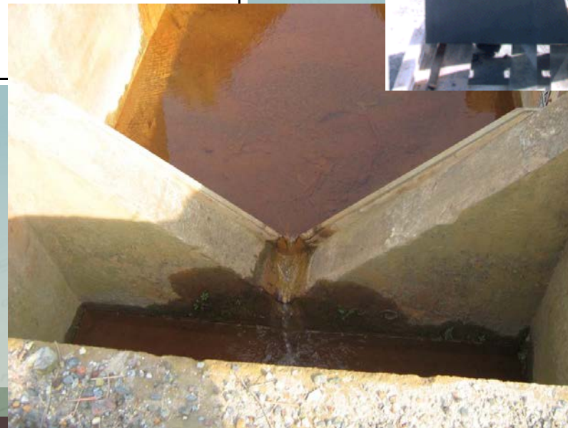
Flow Through a V-Notch Weir
