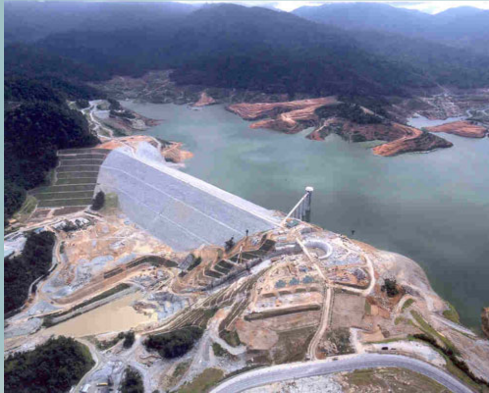
Water Supply Dam ( Sg. Selangor )
