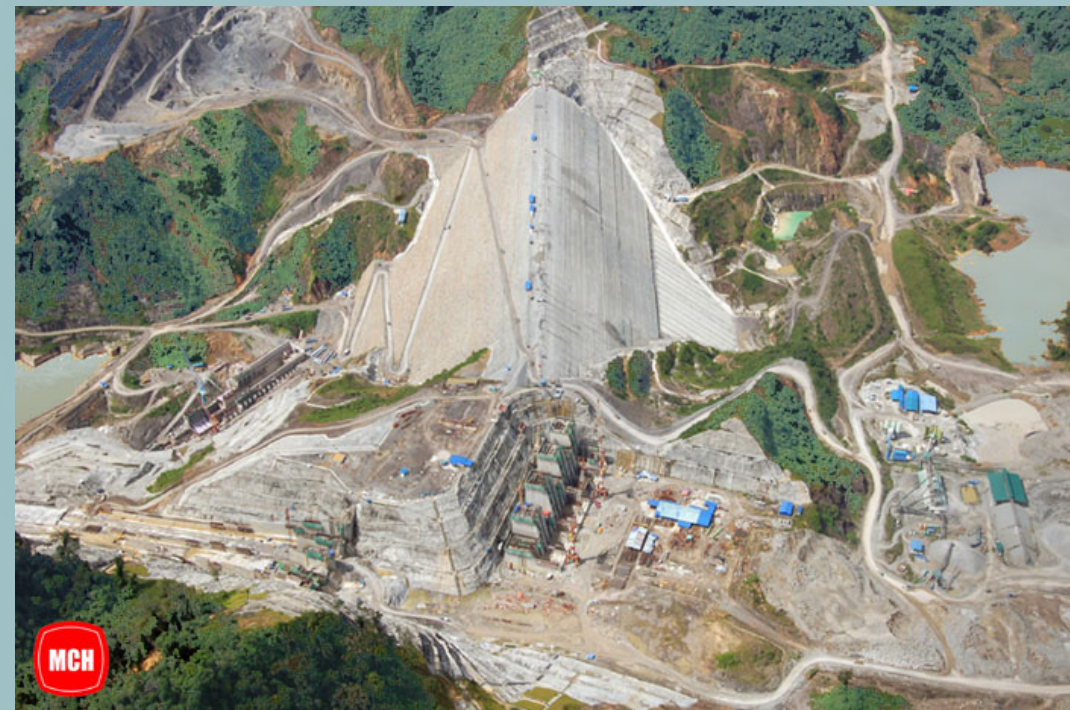
Hydropower Dam - Bakun ( SESCO )
