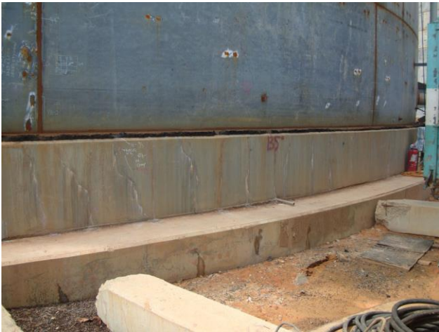
Fig. 3a. Tensile Cracking on Upstand Ring Beam during Hydrotest (9pt, left aligned)
