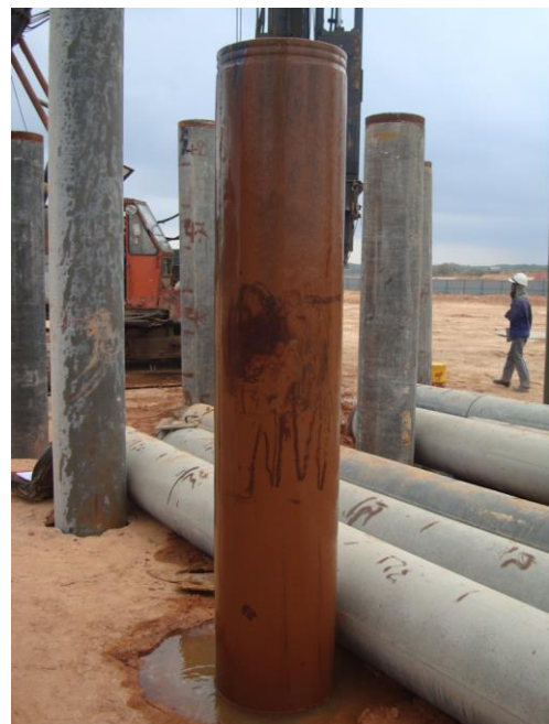
Fig. 1. Water Overflowing in Pile Annulus as Evidence of Excess Pore Water Pressure in the Ground (9pt, left aligned)
