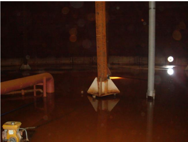
Fig. 3b. Detached Tank Roof Support due to Irrecoverable Bowl-Shaped Tank Raft Deformation after Hydrotest (9pt, left aligned)
