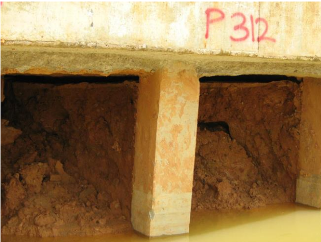
Fig. 4. Settlement of Reclaimed Platform (9pt, left aligned)
